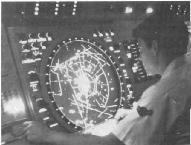
In early 1985, the new AN/GPN-22 precision approach radar, part of the AN/GPN-24 program, stands ready for flight checks on the primary runway at Andersen AFB, Guam. The new radar gave more reliable service because it was simpler to operate and provided more accuracy, greater precision, and more detailed display.
