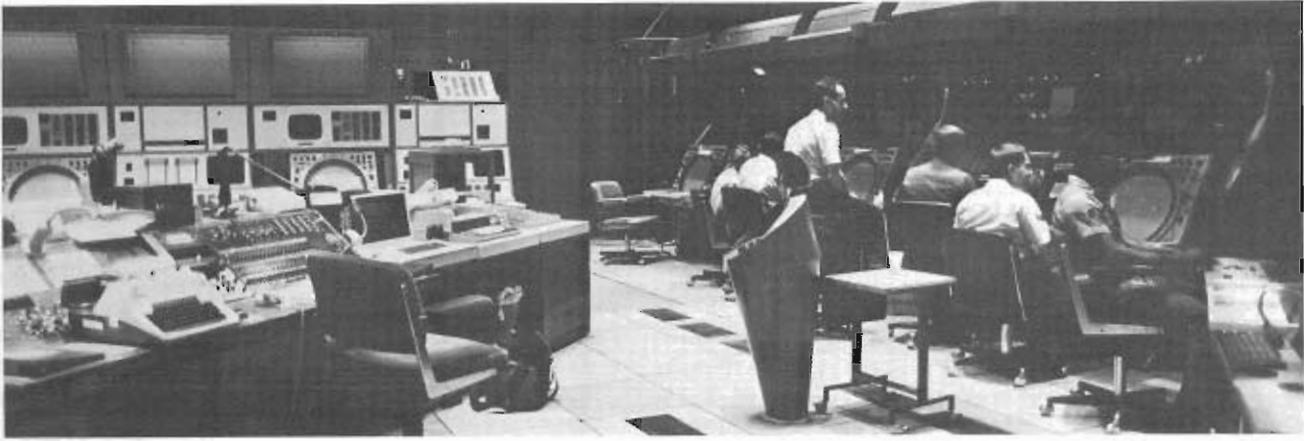
After more than a year of wiring work, the old Siemens consoles, right, were replaced in 1985 by the new OJ-314 consoles, left, at the Berlin Air Route Traffic Control Center, Tempelhof Central Airport. The new console would be used by American, British, and French controllers in accordance with an Allied agreement signed at the end of World War II.
