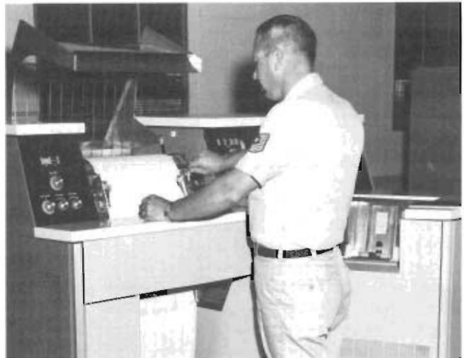
An AFCS airman operates the UNIVAC 1004 high speed printer and reader. This small computer is used in the Automated Weather Network for transmitting weather data.
