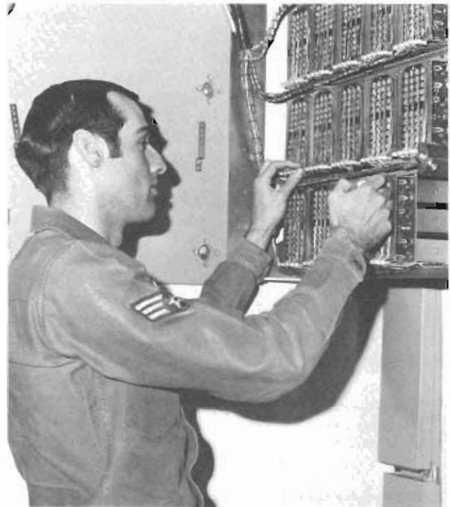
An AFCS airman checks the relays used in a telephone key system. A relay panel such as this one can carry as many as 50 dial or 20 direct lines.
