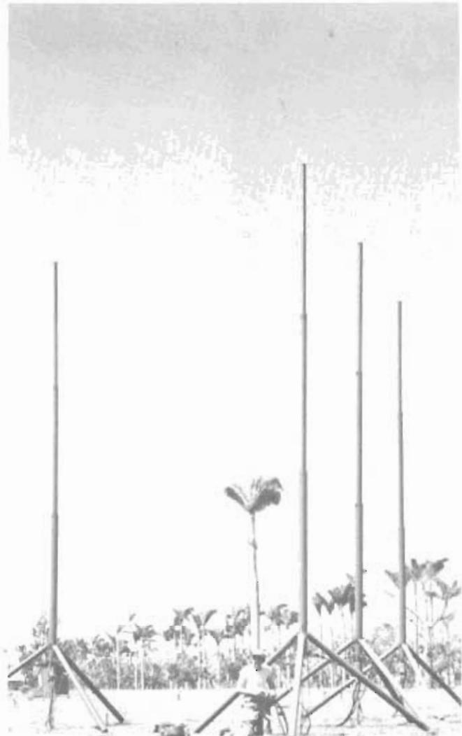
Pictured here is one of AACs's mobile range stations used to broadcast radio beams, which served as highways in the air for Army Air Force planes. These stations enabled the armadas of Boeing B-29 bombers striking Japan to return to bases on pinpoint islands in the vast Pacific in instrument weather.
