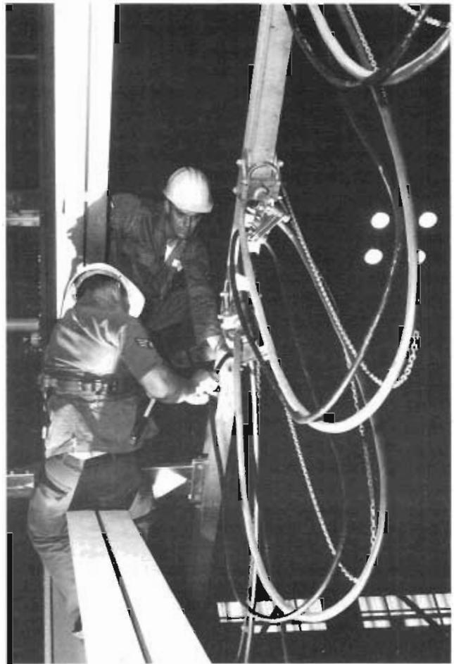
High riggers from the Ground Electronics, Engineering, and Installation Agency install cables on a mobile service tower at Cape Kennedy AFS, Florida, prior to a missile launch.
