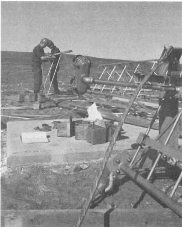
SrA Sid Trekel and A1C Mike Trevizo of the 485th Engineering Installation Group complete the boom section of a heavyweight rotatable log antenna on North Mountain, near Thule AB, Greenland.
