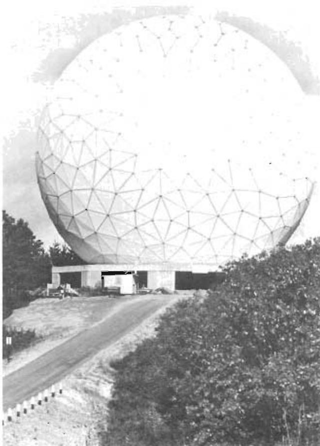
This aluminum and fiberglass radar dome protects a communications and space research antenna in Massachusetts.
