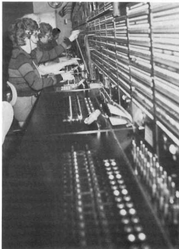
Kelly AFB, Texas, telephone operators operate the old switchboard for the last time. The next day the telephone switching system was replaced by a state-of-the-art digital switching system. This replacement was part of an AFCC program known as Scope Dial, a project to modernize base telephone systems around the world.
