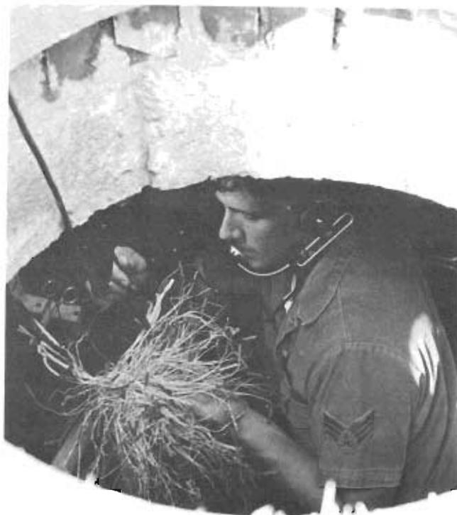
A cable splicer with the 1974th Communications Group works in a manhole at Scott AFB, Illinois.
