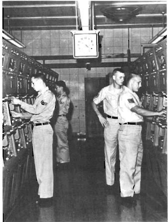
AFCS airmen check equipment in the "Plan 55" Automatic Teletype Relay at Andrews AFB, Maryland. Incoming teletype messages, received at 60 to 100 words per minute are read, automatically "switched" across the center at a rate of 200 words per minute, and sent to the addressee at the speed his equipment will receive it.
