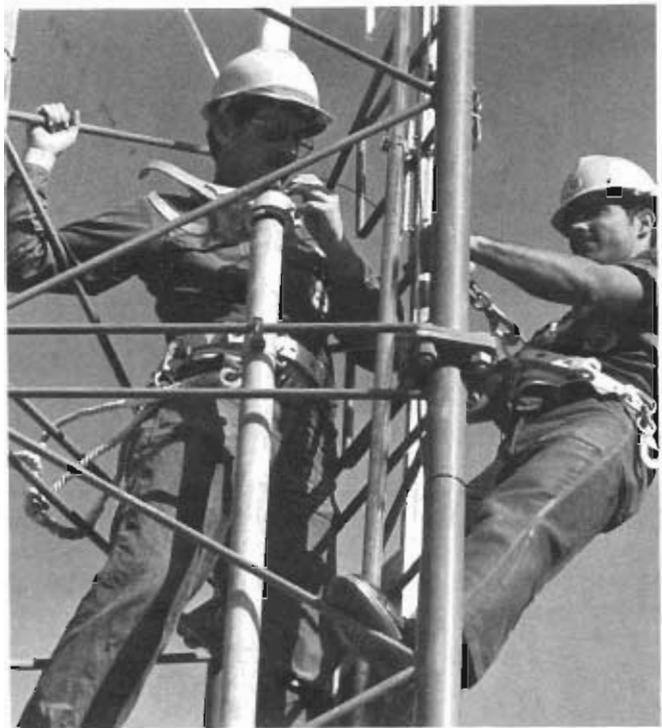
Members of the 1923d Communications Installation Group, Kelly AFB, Texas, install conduit on the glide slope antenna tower. The tower is part of a new electronic system (the GPN-29 solid state instrument landing system) that guides aircraft to the primary landing runway at Holloman AFB, New Mexico.
