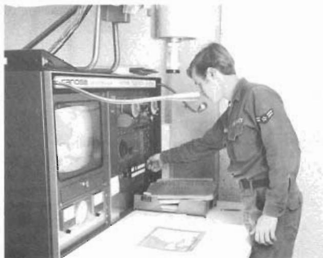
An AFCS airman adjusts the focus on a closed circuit television system in a base weather station.
