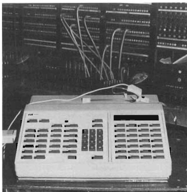
The cumbersome 1938 vintage R-7D switchboard, in the background, one of the oldest in the US Air Forces in Europe command, and the new switchboard console of the DMS-100/200 illustrate the conversion from the old to the new in voice communications at the 2186th Communications Squadron at Torrejon AB, Spain.
