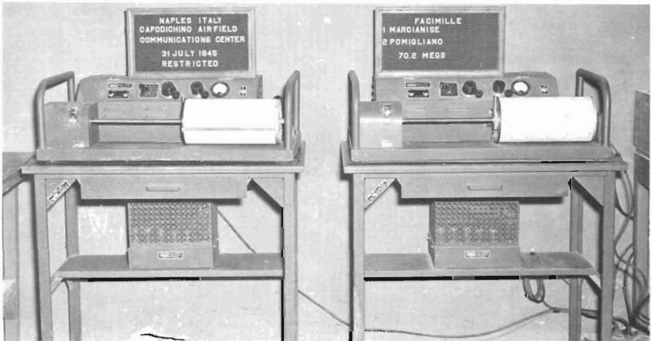
Facsimile transmission was first used in AACCS in 1943 to relay weather maps. This system worked over ordinary telephone lines. Using 96 lines to the inch, it took 20 minutes to transmit a standard map covering the approximate area of the continental United States. The machines shown here were employed at Capodichino Airfield, Naples, Italy.
