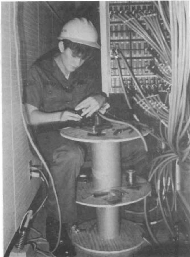
A1C Sharnee Riley, radio team member, 1837th Engineering Installation Squadron, uses an Amphenol "Amp-Champ" crimper to terminate a connector on one of the multitude of 25-pair cables installed at the control site as part of the Scope Signal III installation at Clark AB, Philippines. Scope Signal III is the program to modernize Giant Talk, the Strategic Air Command's world-wide command and control network. The station at Clark was the first Air Force-installed station to come on line.
