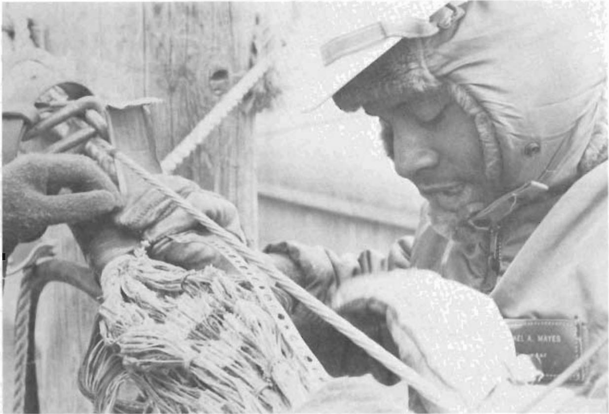
In subfreezing temperatures, a member of the 1839th Engineering Installation Group fastens a 100-pair bridge to a 400-pair cable during a cable expansion project at Incirlik AB, Turkey.
