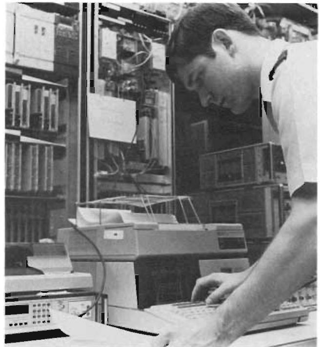
2LT Norman Howard, 1842d Electronics Engineering Group, verifies automated procedures on the prototype digital microwave radio system. This installation supports the Japan Reconfiguration and Digitization program. These radios are now being installed at various sites in Japan and the automated tests are used to verify system performance and accomplish test and acceptance in the field.
