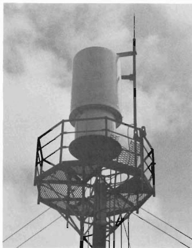
In March 1985, AFCC installed a prototype of a TACAN antenna (AN/GRA-121) with a heated radome at Shemya AFB, Alaska. The heat made the antenna, used for enroute and terminal service, invulnerable to blowing snow and ice buildup.
