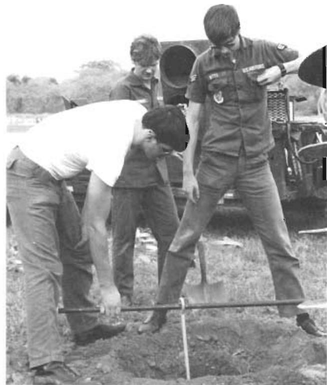
Three AFCS airmen install a ground rod for a mobile control tower.
