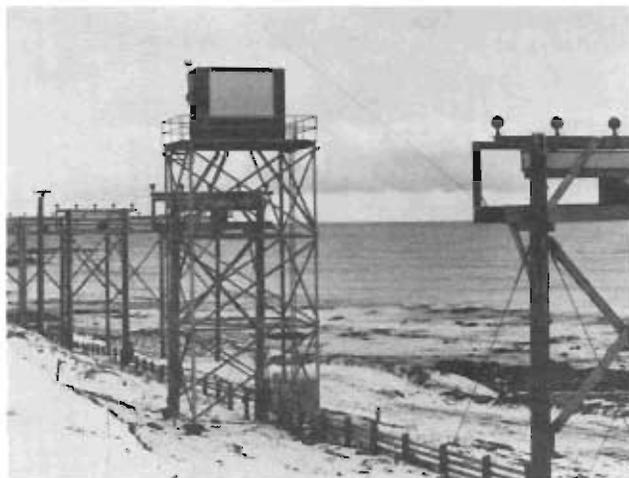
This 2-degree azimuth facility on its 30-foot tower was part of the microwave landing approach system at Shemya AFB, Alaska.
