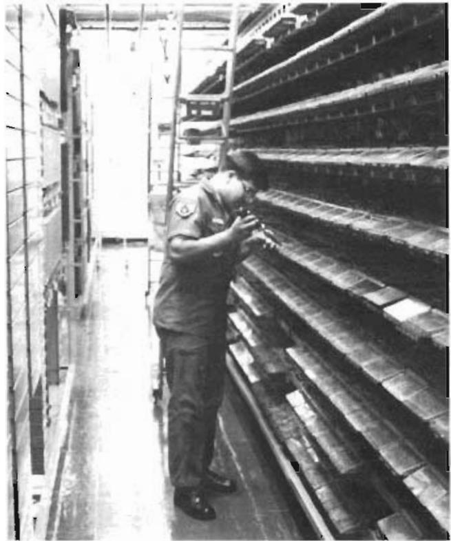
An AFCS technician performs preventive maintenance on the Norton AFB, California, telephone switchboard mainframe.
