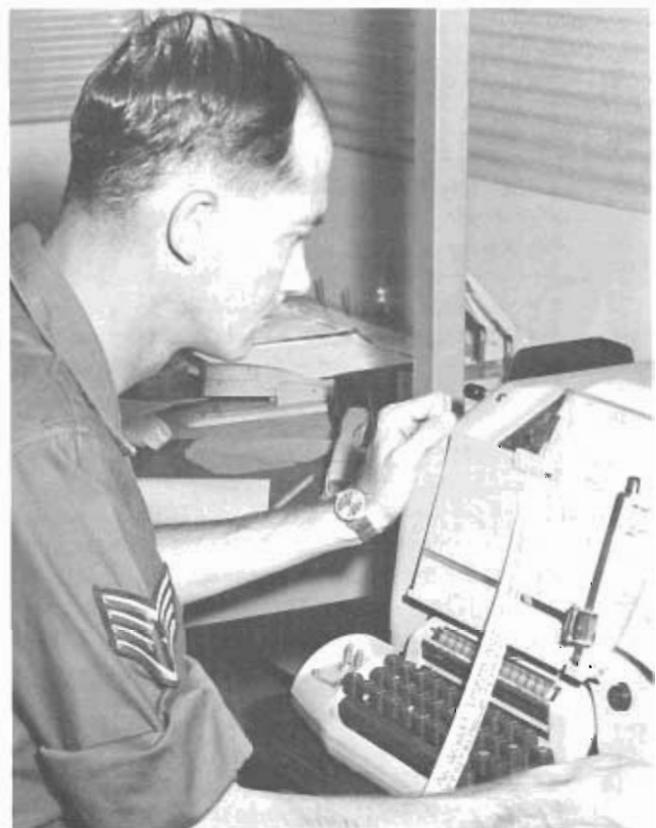
Introducing equipment that would transmit and receive messages in a variety of formats was one of the advanced features of the AUTODIN network. Here, an airman prepares a message on paper tape.
