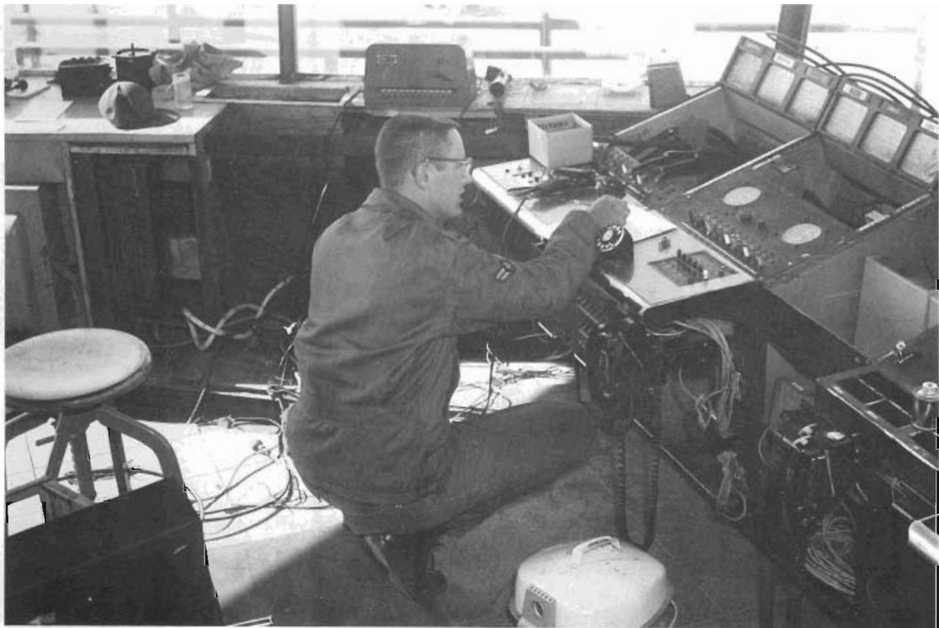
A control tower is just as much an integral part of the Air Force as an airplane. Here, an AFCS technician rewires the control tower as part of the continual rehabilitation, modification, and maintenance efforts to ensure adequate support of aircraft.
