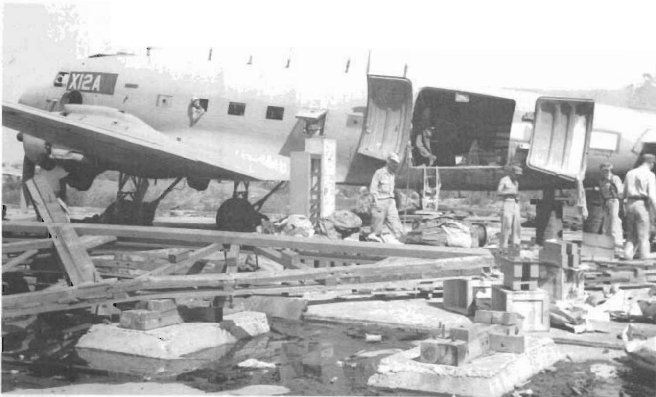
One hour after landing at Atsugi Airfield, near Tokyo, Japan, the AACS transmitter plane, a radio equipped C-47 (Gooney Bird), similar to the receiving station plane shown above, was on the air sending out signals to Okinawa. There was only one hitch in operations, when on the second day rains and motor traffic shorted out the five lines which ran to the receiver plane. Damage suffered by the field can be seen in the foreground.
