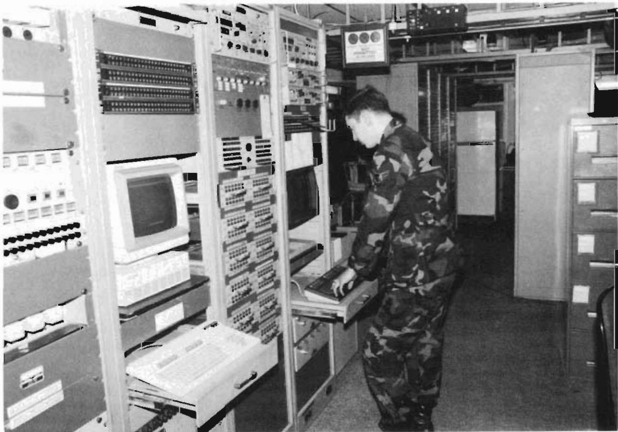
A1C Mark Williams checks the status of Digital European Backbone remote unmanned sites using transmission monitoring and control equipment.
