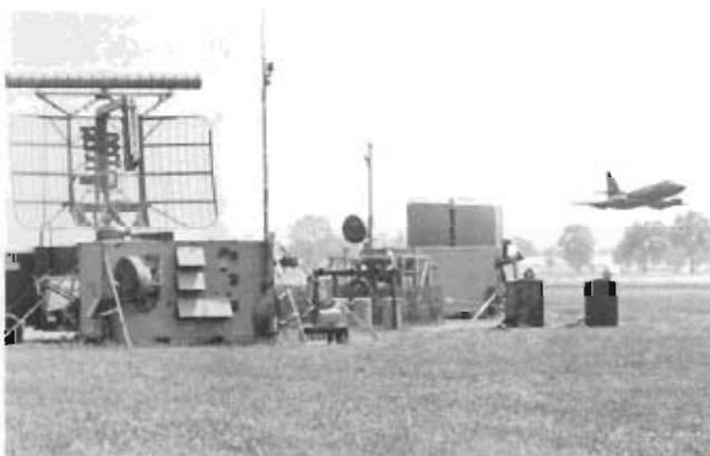
Mobile air traffic control and navigation equipment such as this AN/TPN-19 allowed AFCS to direct aircraft traffic in a variety of contingency and emergency situations.
