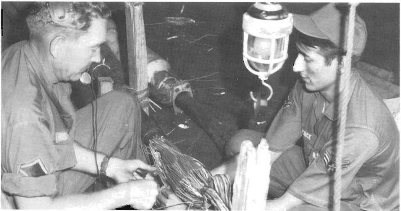
Damaged circuits required that AFCS technicians be constantly ready to provide repair services to insure continued operation of important communications facilities.
