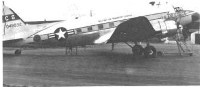
During the 1950's, AACS employed various types of specially configured aircraft to flight test and calibrate navigational aids and flight control facilities. The AC-47D pictured here remained active in the command's inventory until 1962.
