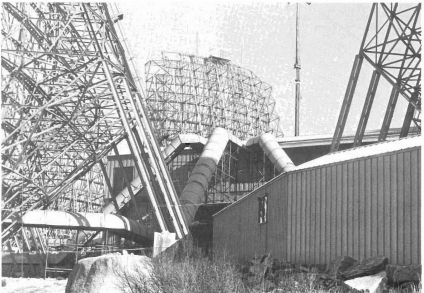
Tropospheric scatter antennas like these operated by the 2181st Communications Squadron at Mt Vergine, Italy, provided a vital link in the communications network in Europe.
