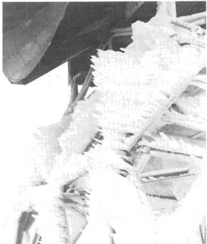
Ice and snow driven by the severe arctic winds accumulate on antenna supports at Cape Lisburne AFS, Alaska.
