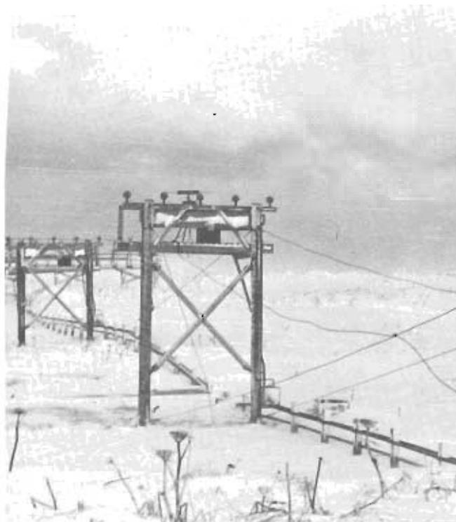
The Alaskan earthquake damaged or destroyed much of the state's communications facilities, including the air traffic control approach lights in this picture.
