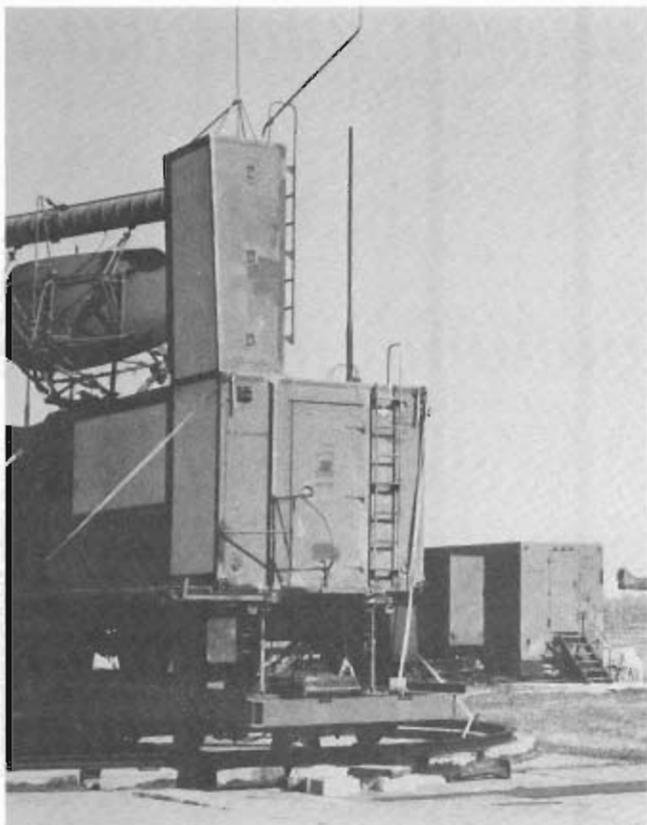
In the fall of 1985, a 1st Combat Communications Group AN/MPN-14 mobile air traffic control radar unit and crew supported Canadian forces at Baden Soellingen, West Germany. The radar set is a complete ground control approach facility used as an air traffic control center.
