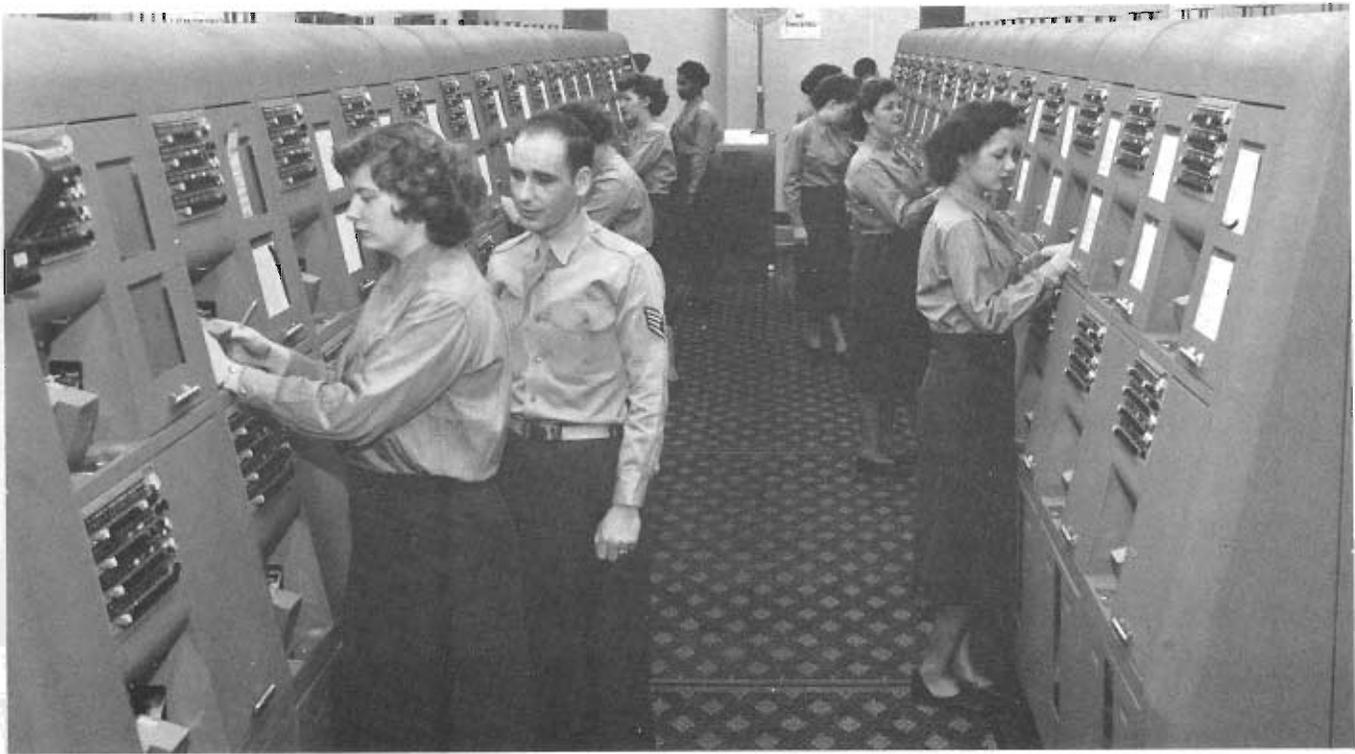
The Air Force's nationwide, push-button communications system was inaugurated on 9 April 1951. The high speed telegraphic communications network linked 179 stations in the United States. Five switching centers replaced the 28 centers of the previous system. The Air Force leased the system from the Western Union Telegraph Company, but staffed it with its own operators. The five centers were the continental portion of the Air Command Communications Network.
