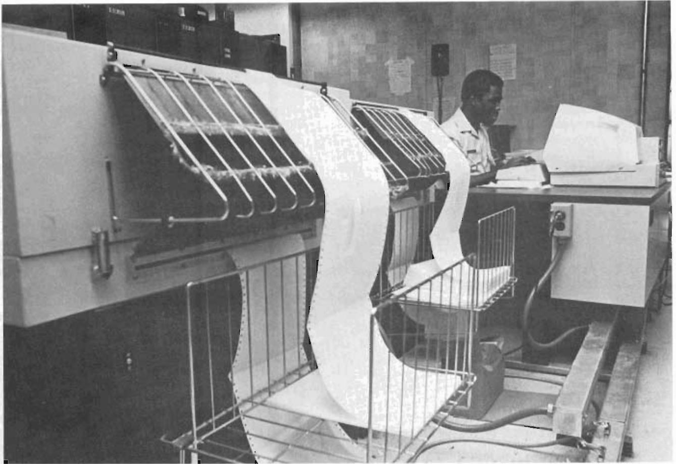
Console operator SSgt Clifford R. Liggins gives instructions to the Automated Message Processing Exchange equipment, in background, to direct the flow of messages through the 600-line-per-minute printer.
