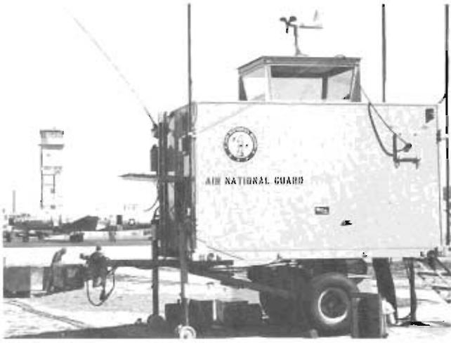
The remodeling of the Mountain Home AFB, Idaho, control tower necessitated the use of a mobile air traffic control tower. This equipment was deployed and setup by Air National Guardsmen from Washington.
