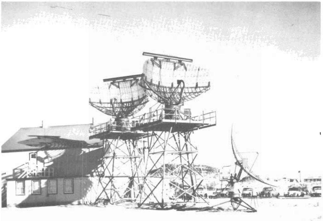
In defending the United States from enemy air attack the man on the ground has become equally as important as the aircrew. Ground control intercept radars such as these are essential in directing pilots to the exact location of their target, whether in training or combat.
