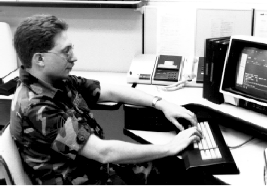
The telephone switching systems supervisor programs Scope Dial features into the DMS-100 telephone switch.
