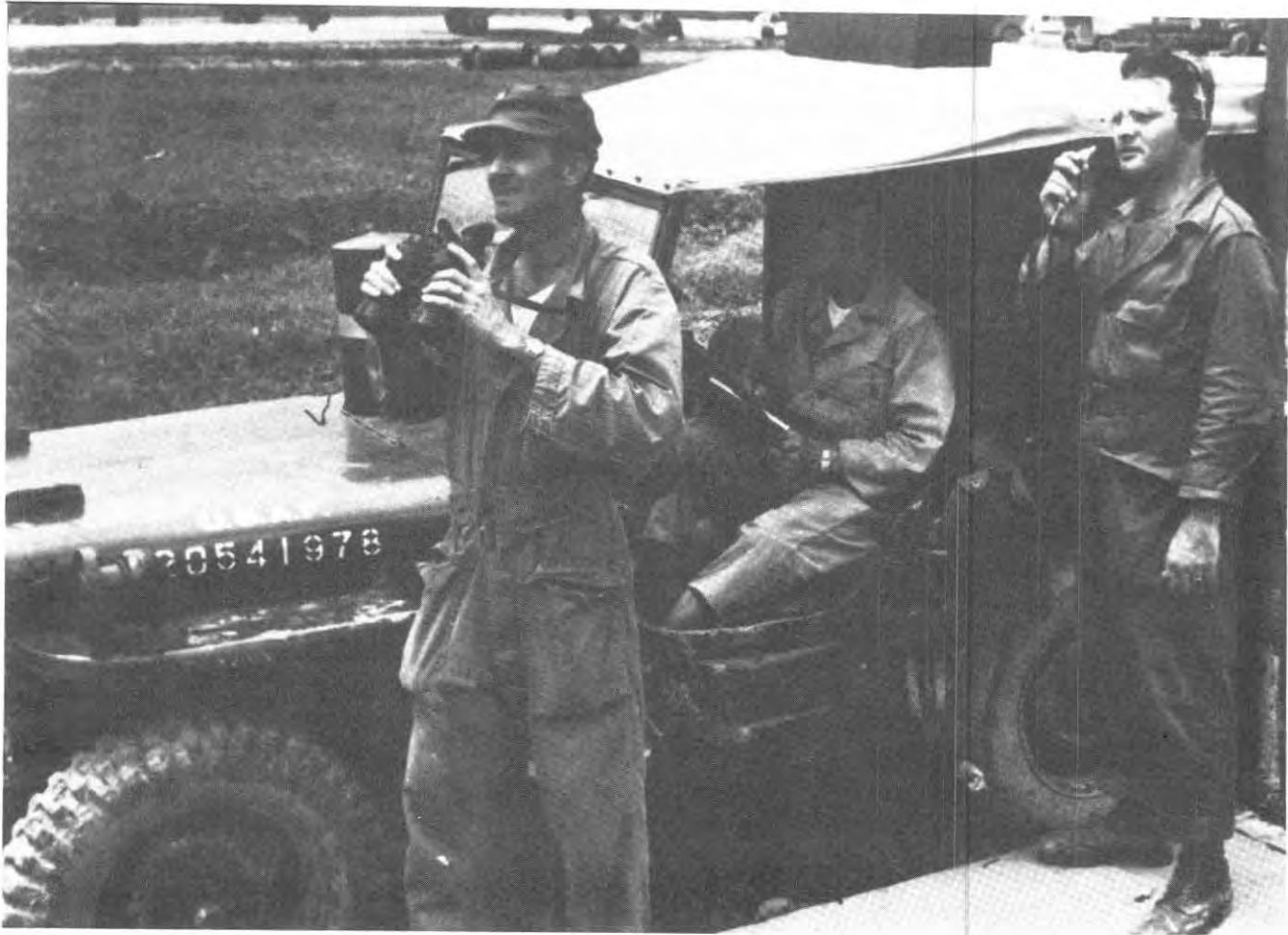
AACS detachments were operating at Pusan, Taegu, and Pohang, Korea, within a week after President Truman authorized American military involvement. The first unit to go into action was this radio jeep which served as a control tower at Pusan.
