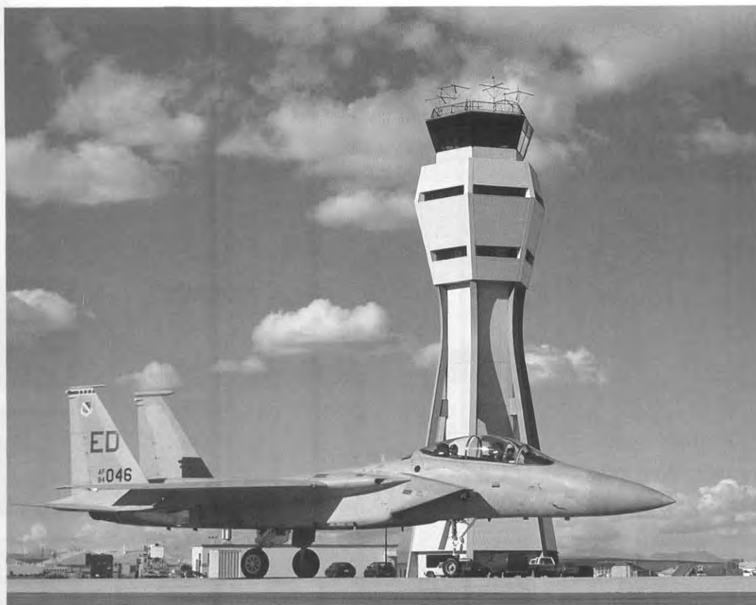
An F-15 Eagle taxis past the new air traffic control tower at Edwards AFB, California. The ten-story structure can withstand winds of up to 120 knots and earthquakes measuring 6.0 on the Richter scale.
