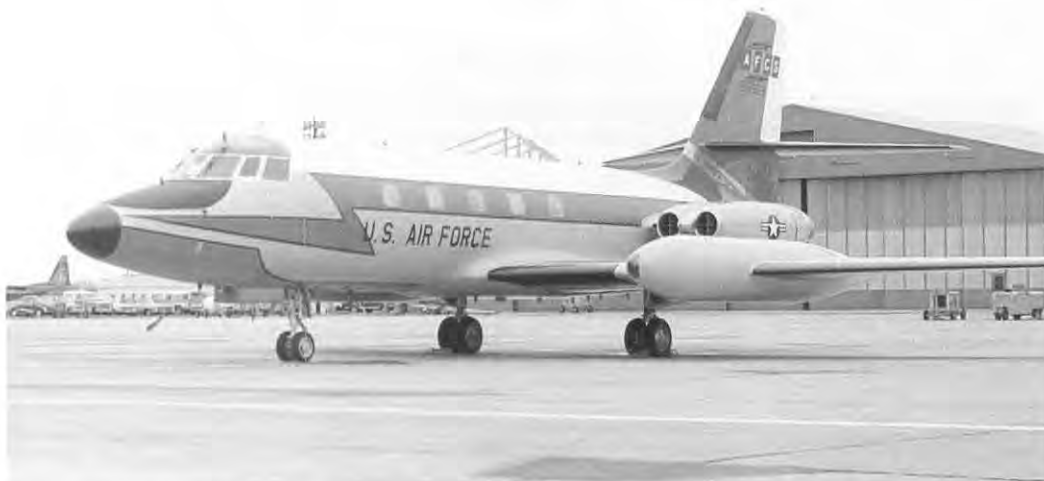
The Air Force Communications Service utilized specially configured C-140s, like this silver and bright red one, to check Air Force air traffic control and air navigational aids for accuracy and efficiency at air bases around the world.
