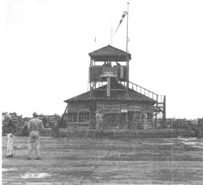
The first control tower in Japan, after the war, was operated by a unit of the 68th AACS Group, which is now the 1956th Communications Group. Initially, the Japanese had used a wooden platform on top of the base operations building; however, the AACS 7th Wing, needed a better structure to protect their radio equipment. The tower was built by the Japanese within eight hours vice the normal two days.
