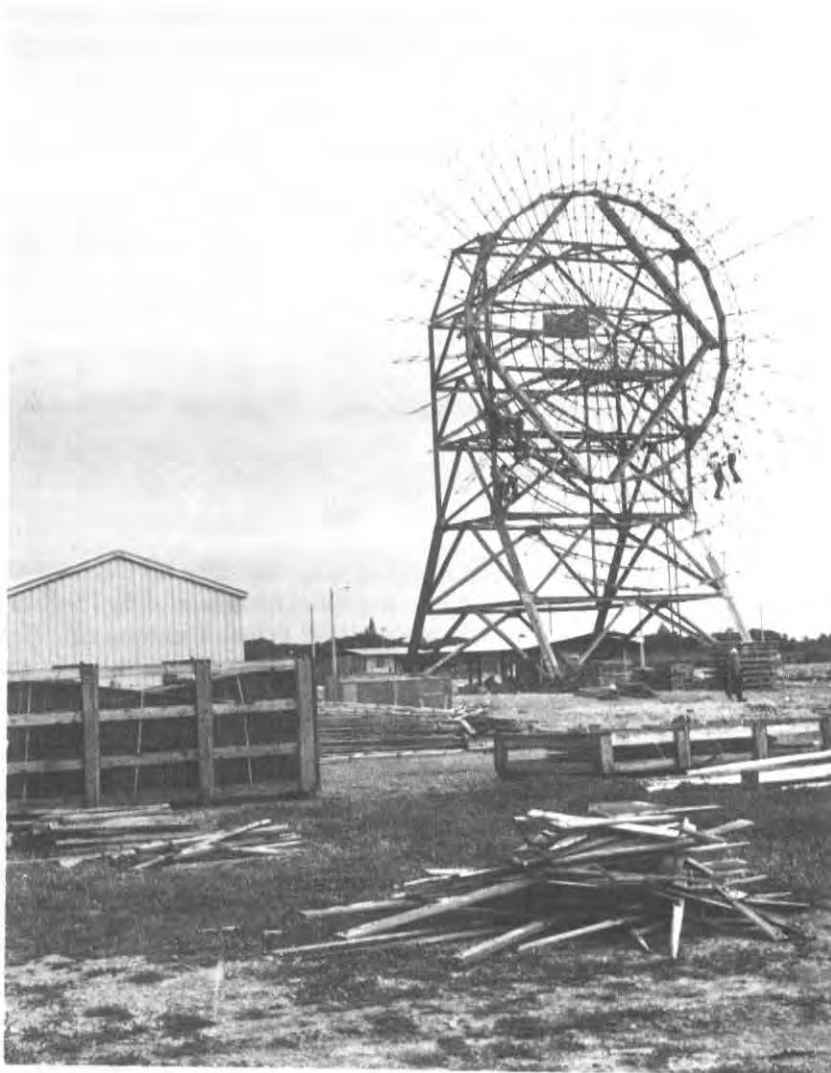
AFCS personnel work on a 60-foot parabolic antenna at Ko Kha, Thailand, part of the extensive communications network in south-east Asia, created in response to the Vietnam conflict.
