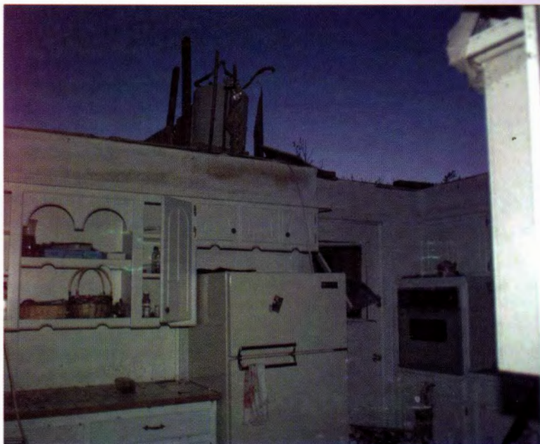
Inexplicable — even though the family kitchen remains standing with typical household items still on their shelves, the roof and walls of this Oklahoma City home were completely sheared off and spewed out as loose debris in the surrounding area.
